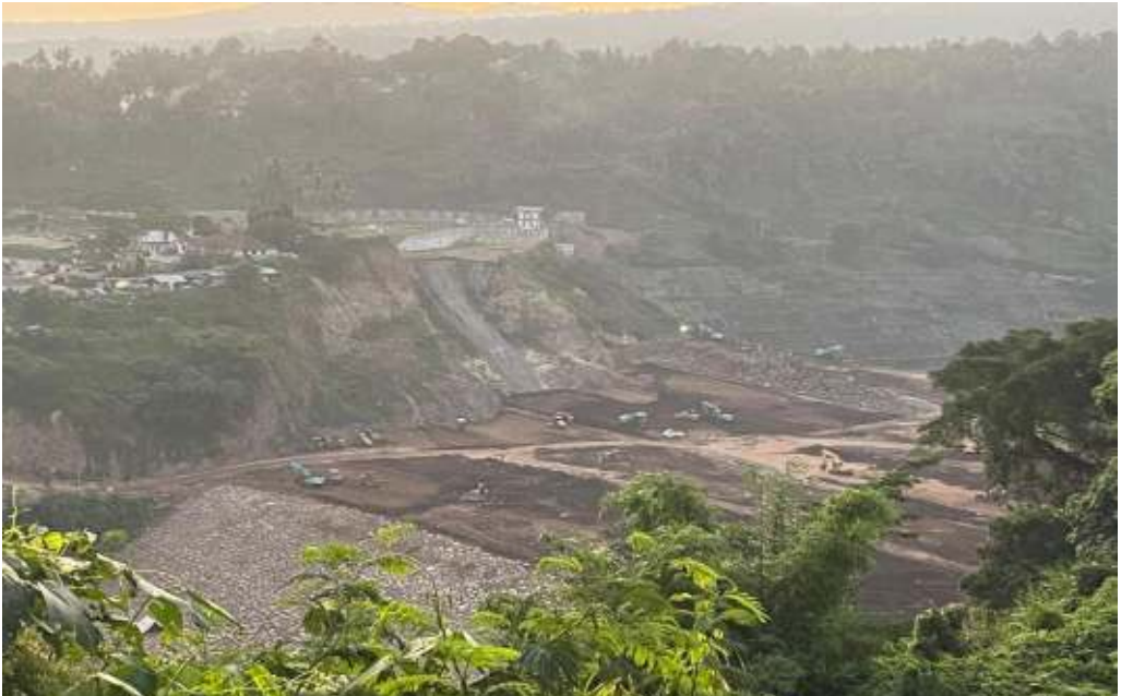
(SP Mataram Documentation, Condition of Meninting Dam Construction on June 12, 2024, the form of the reservoir pond is still not visible)
